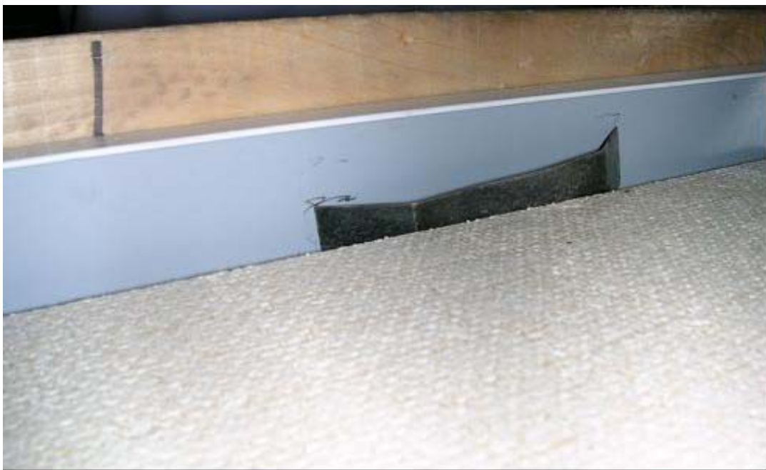
Figure 2–29. Panel perimeter spring clips in ceiling system CS1.
